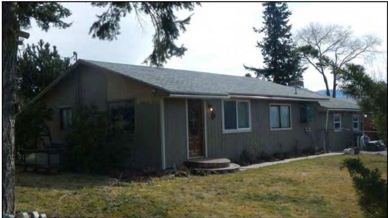
Figure 38. Residence at 5 South Stark Avenue, East Wenatchee. View to the southeast.
