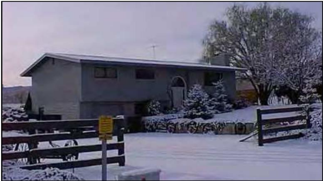
Figure 16. Residence at 3780 Grant Road, East Wenatchee. View to southwest.
