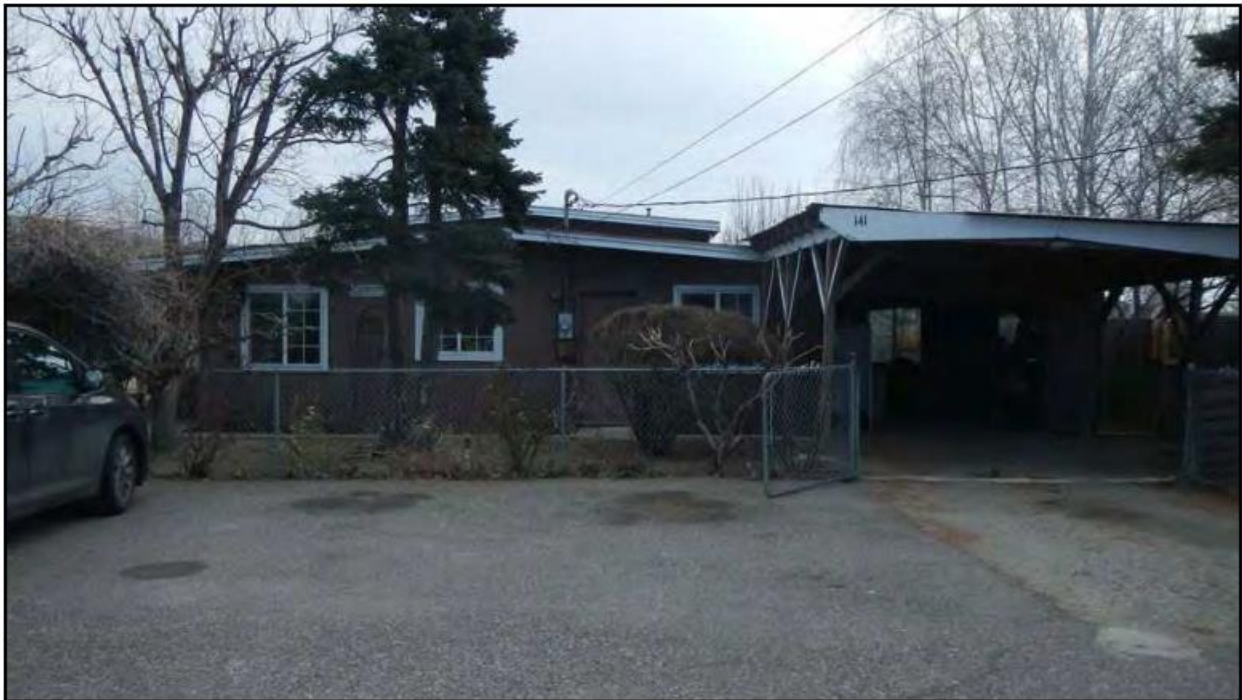
Figure 35. Residence at 141 South Texas Avenue. View to the southeast.
