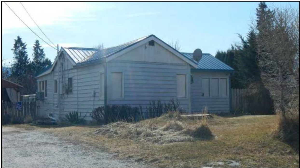
Figure 23. Residence at 50 South Union Avenue, East Wenatchee. View to south-southwest.
