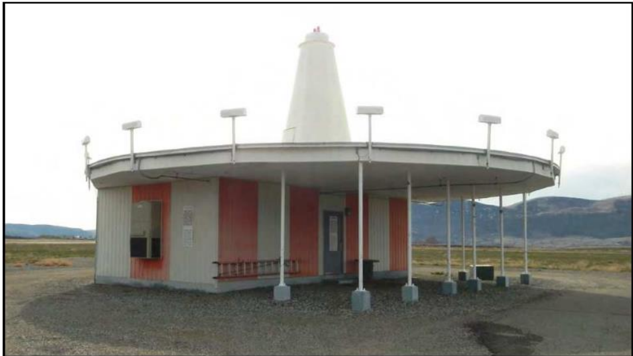
Figure 45. Very High Frequency Omnidirectional Range Facility at Pangborn Memorial Airport. View to southeast.
