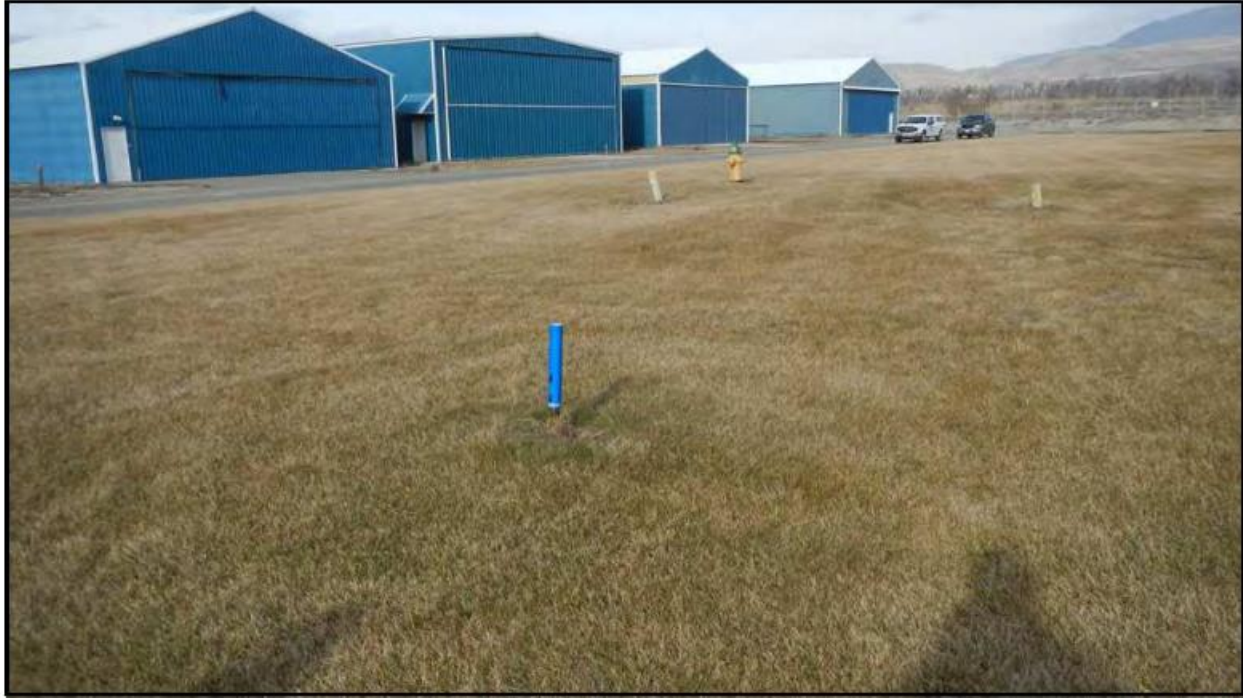
Figure 8. Overview of Project Component 09/Executive Hangars.
