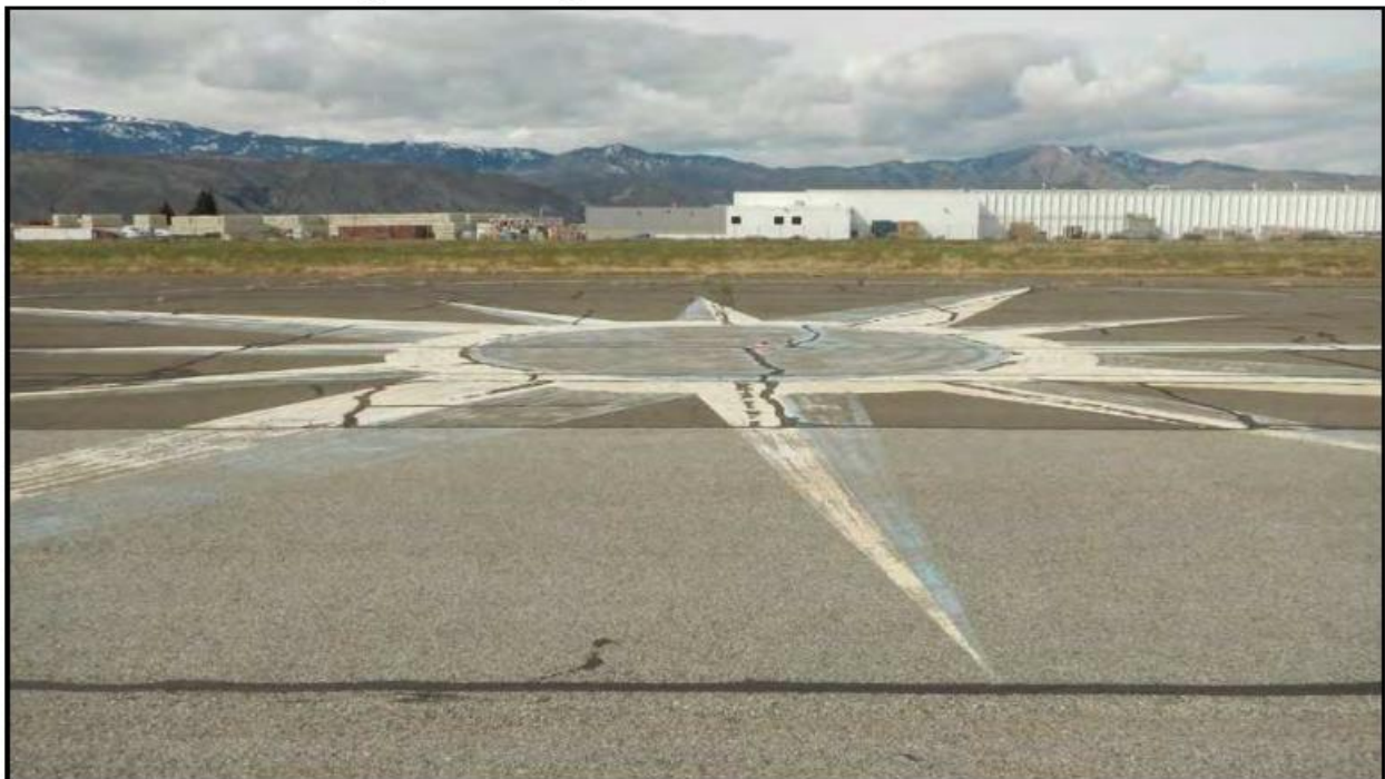
Figure 50. Pangborn Memorial Airport – Taxiway B. View to west, overlooking compass rose.
