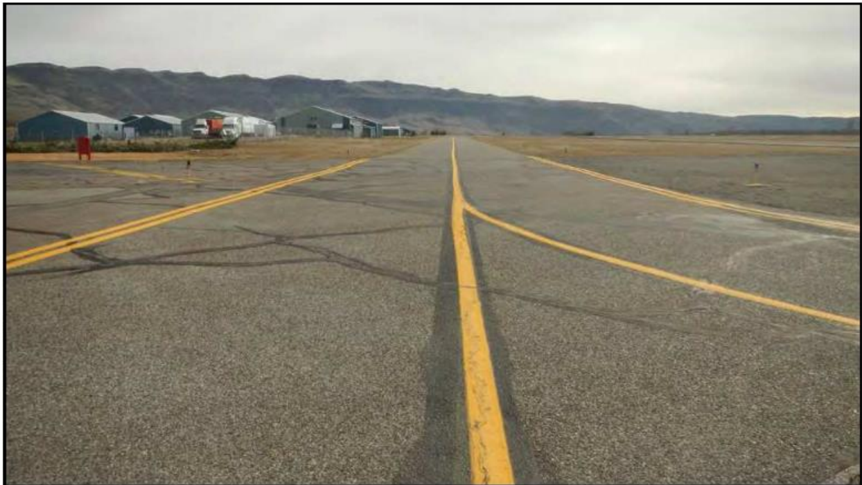
Figure 52. Pangborn Memorial Airport – Taxiway F. View to east.
