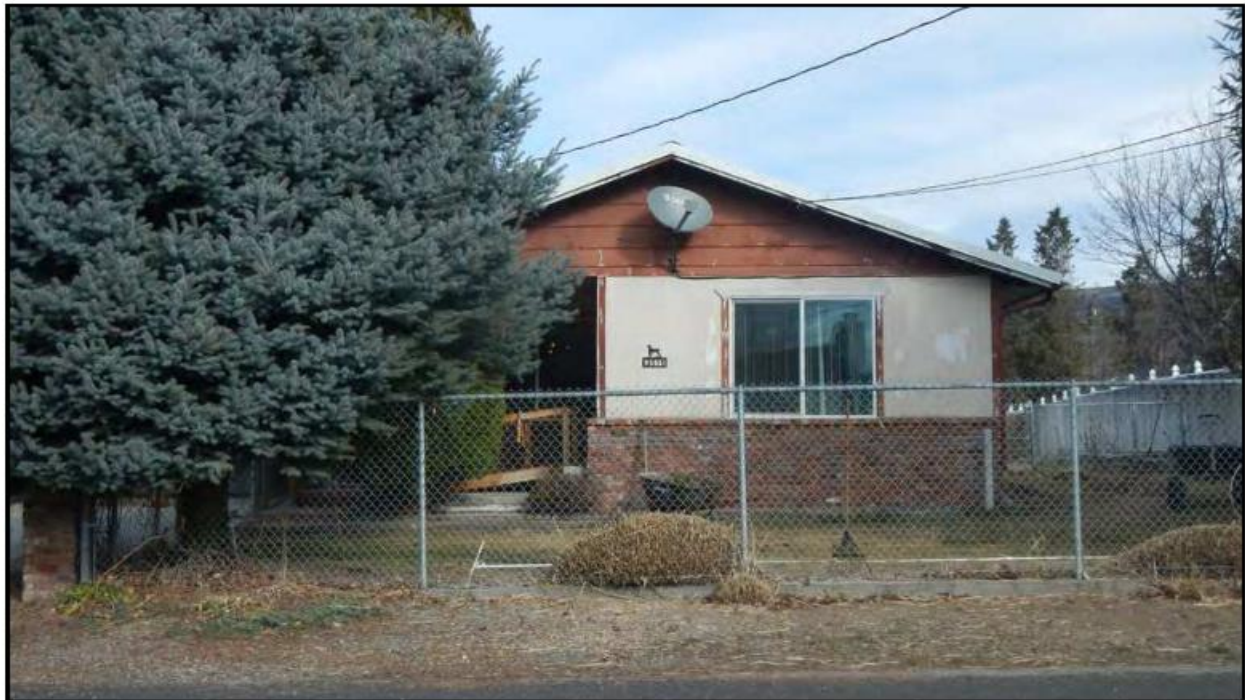
Figure 28. Residence at 3111 Airway Street SE, East Wenatchee. View to the north.
