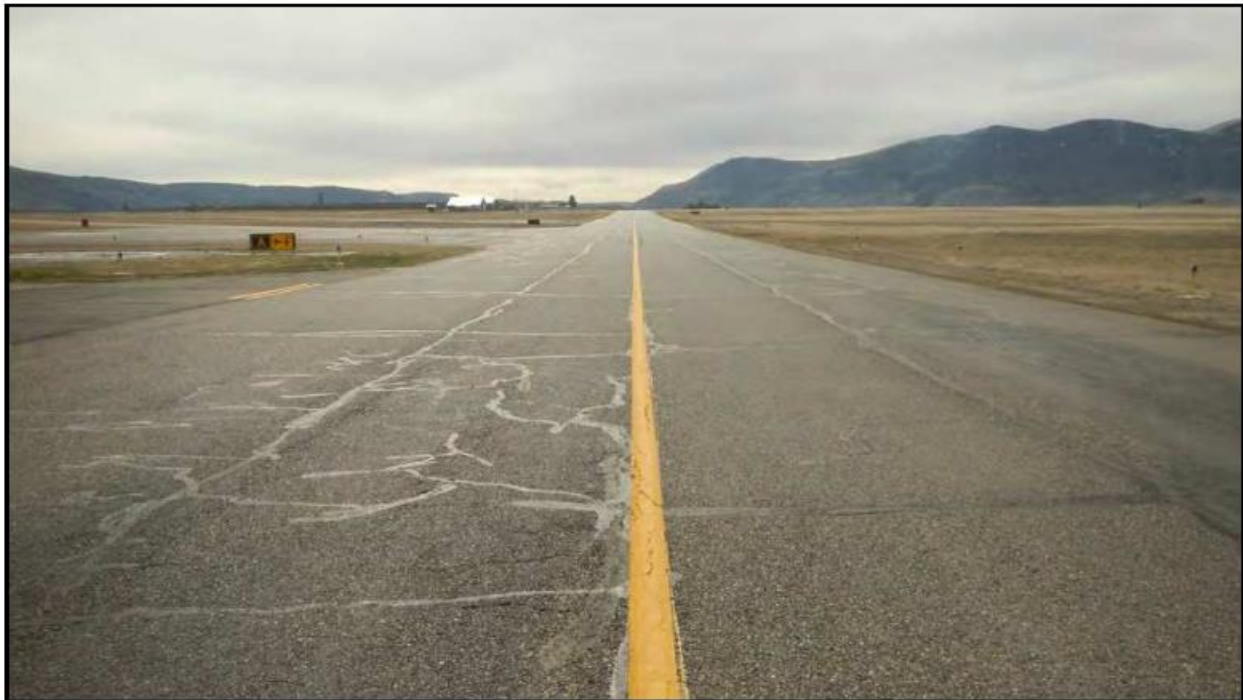
Figure 49. Pangborn Memorial Airport – Taxiway A. View to southeast.
