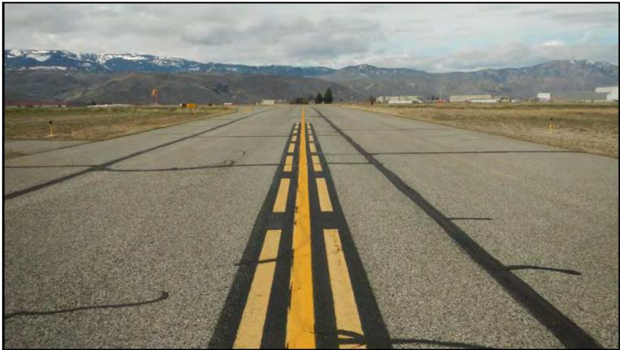
Figure 51. Pangborn Memorial Airport – Taxiway C. View to southwest.
