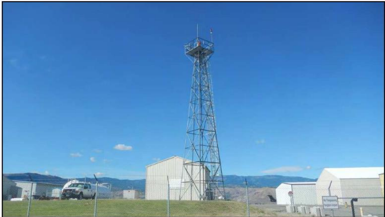
Figure 43. Pangborn Memorial Airport – Beacon Tower. View to west.
