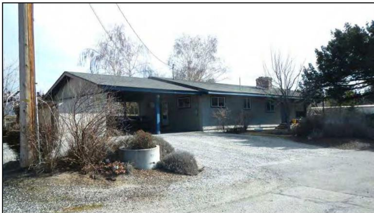
Figure 25. Residence at 39 South Union Avenue, East Wenatchee. View to the east-southeast.
