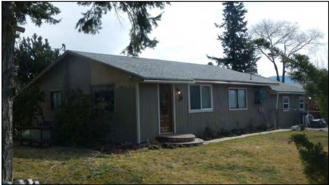
Figure 38. Residence at 5 South Stark Avenue, East Wenatchee. View to the southeast.
