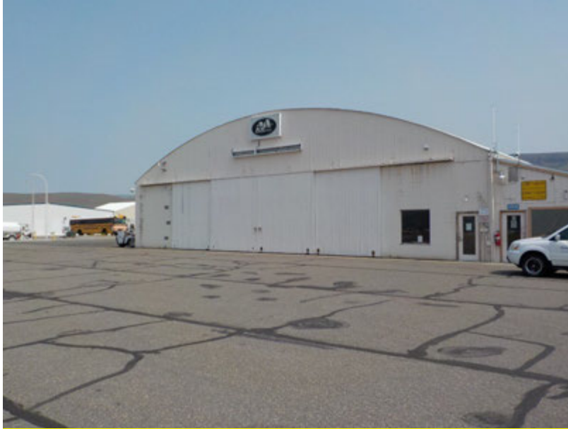
Southwest side view of GA Terminal hangar (looking north).
