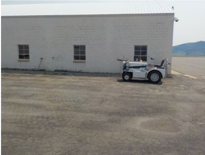
Location of USTs near west corner of GA Terminal Building.
