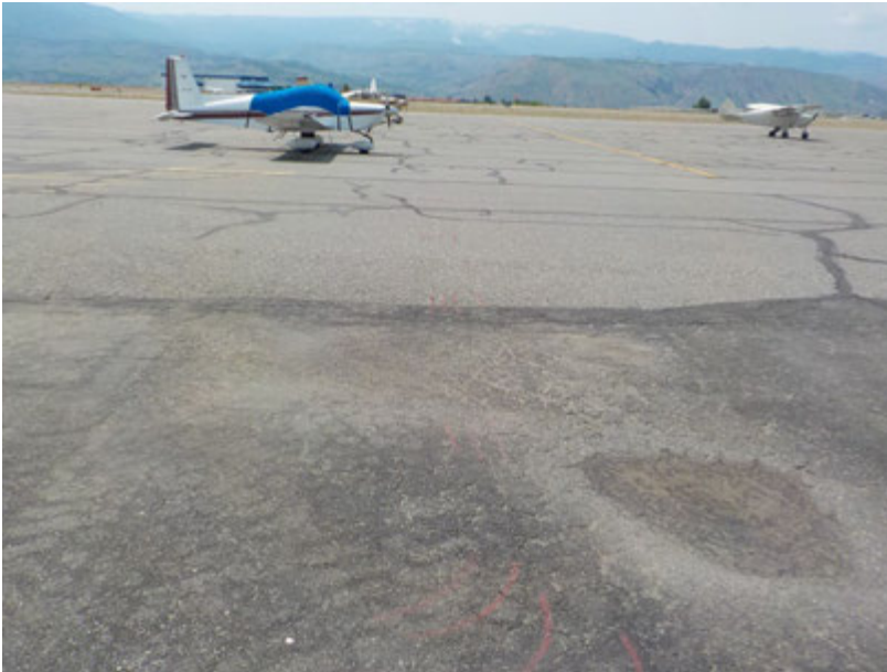
View of Airport apron on adjacent property to the south.
