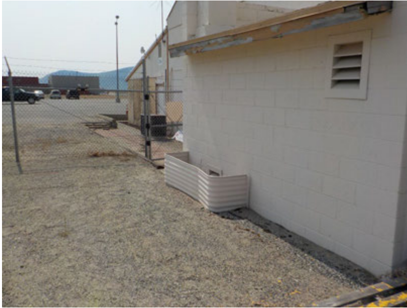
View of building addition on northwest side of GA Terminal Building.
