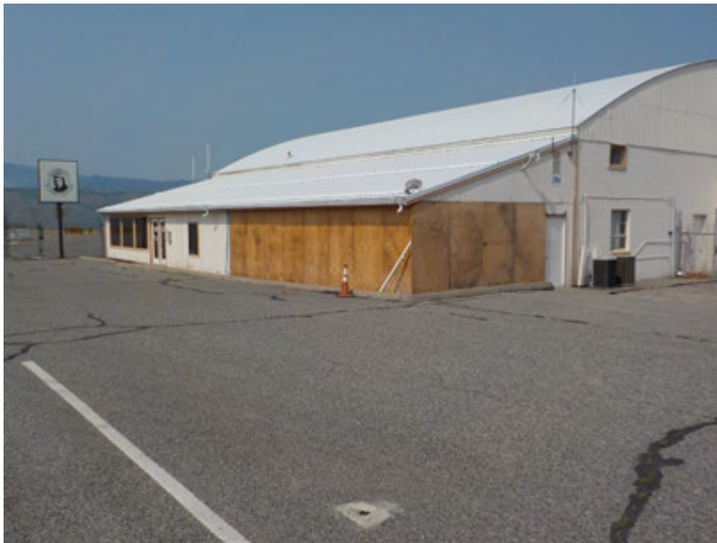
View of GA Terminal southeast building addition (looking south).
