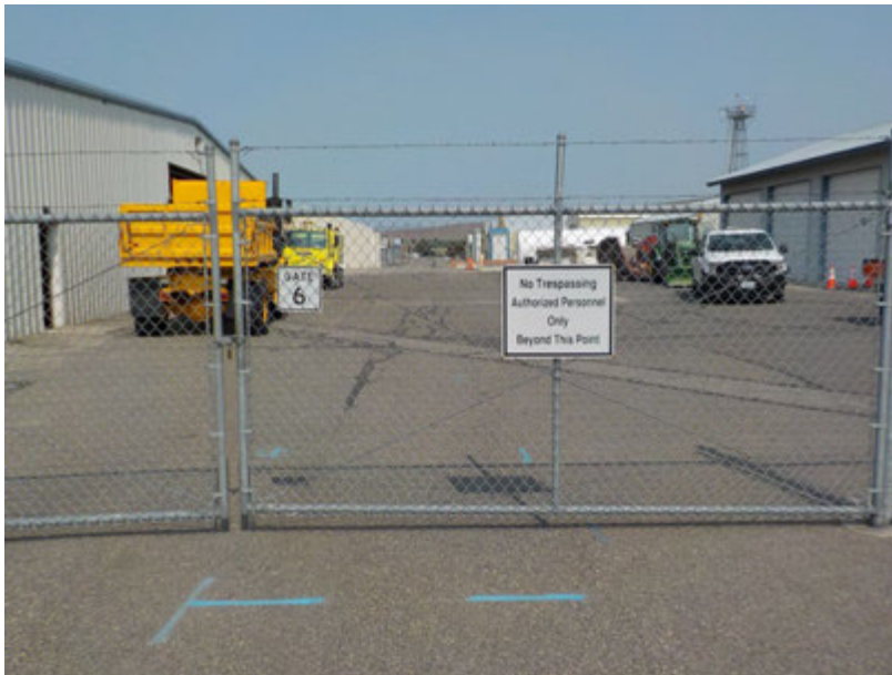
View of Airport maintenance facility north of subject property (looking northwest from subject property).
