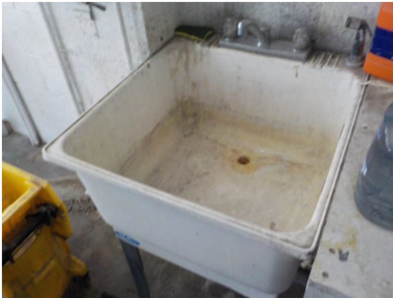
View of utility sink inside hangar.
