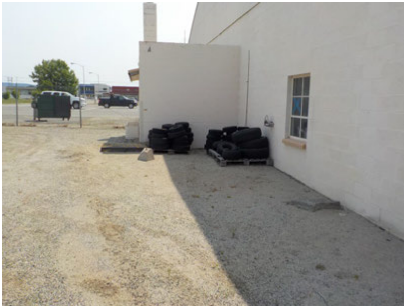
View of heating oil UST location near northeast side of GA Terminal Building.
