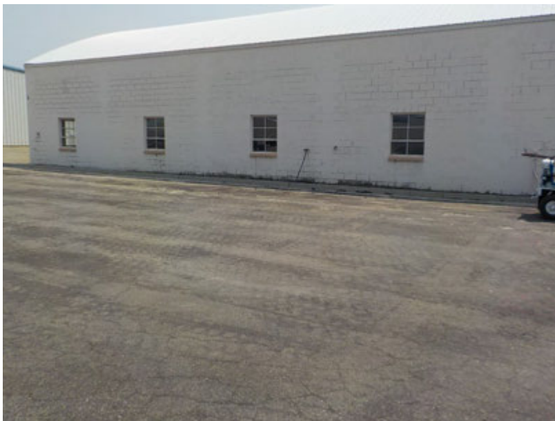
View of northwest side of GA Terminal Building hangar area.
