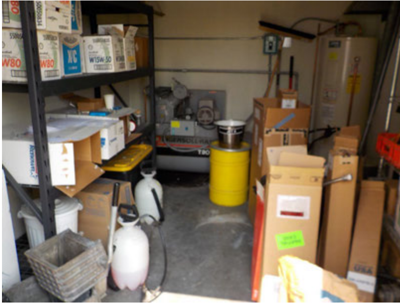
View inside of northwest building addition.
