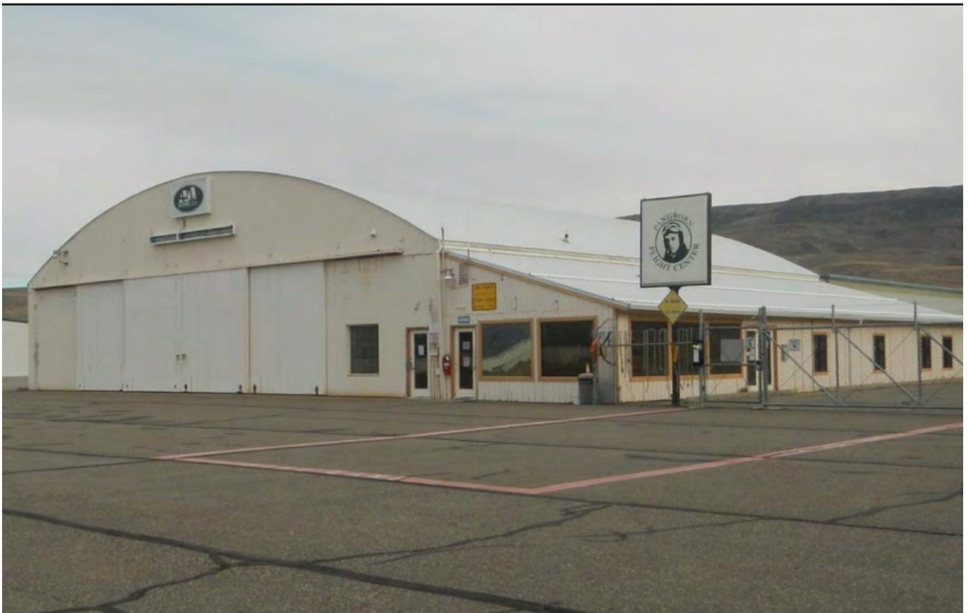
Figure 1-3: Looking northeasterly at the front of the existing GA Terminal building.
