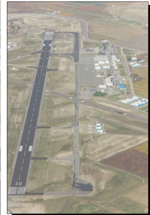
LOOKING NORTHWEST AT RUNWAY 12-30 AND TAXIWAY A [PHOTO DATE: 11-8-16]
